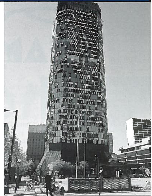
The Bank One building sustained heavy damages
