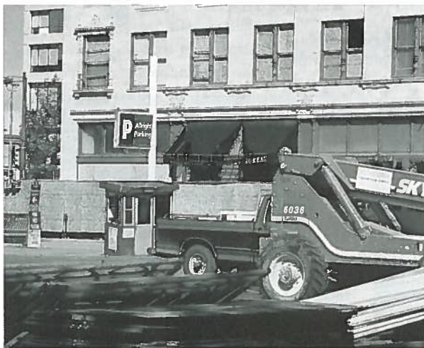
Fort Worth CVB undergoes repairs.
