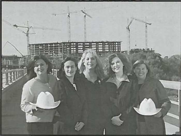
National Sales Managers for Gaylord Opryland Resort & Convention Center (l-r) Wendy Ezernack, Amy Smith, Michelle Carter, CMP, CHSP, Kerri Atterberry and Pam Altman stand in front of the on-going hotel construction project on the shores of Lake Grapevine. The sales staff also includes Kristen Harris (not pictured).
